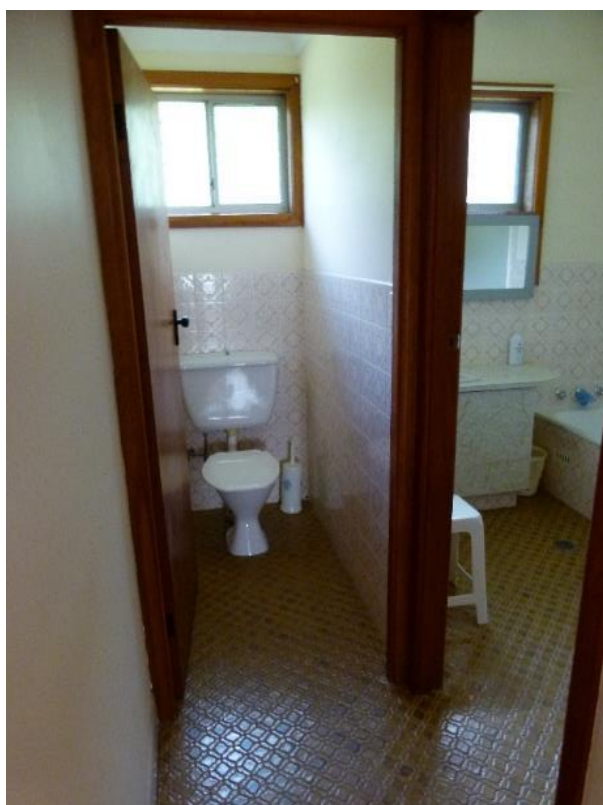
Figure 12: Toilet and bathroom
